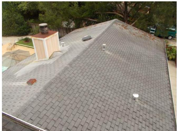
Shingles around the chimney have been replaced and when new shingles are installed it would be a good time to replace chimney flashing and damaged siding.
